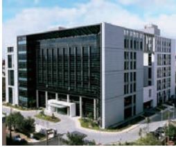
Taoyuan Technology Center (Green Building)
